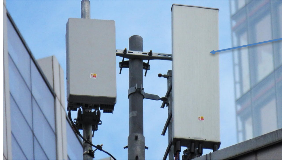
Active Antenna Units RRU integrated with antennas
